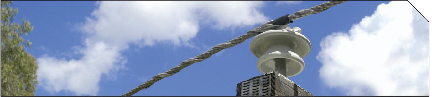
Side Ties are designed and manufactured to secure conductors to the side groove of the insulator.
