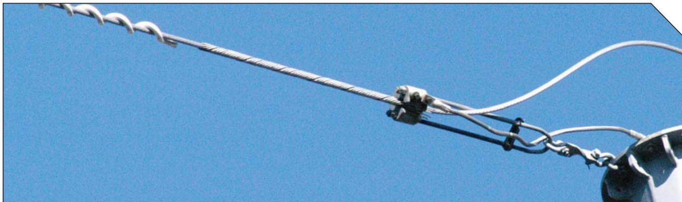
The Fiberlign Deadend is designed to terminate Optical Ground Wire (OPGW) while minimising any compression stresses that may be transferred to the core or optical elements within. The combination of retaining rods, wedge and housing distribute axial and compressive loading over a large area of the OPGW cable. Left-hand or right-hand lay style is provided to suit left-hand or right-hand lay OPGW respectively.
